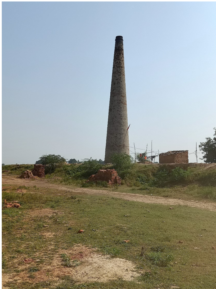
Image 33 : A Brick Kiln As Seen During The Field Survey
