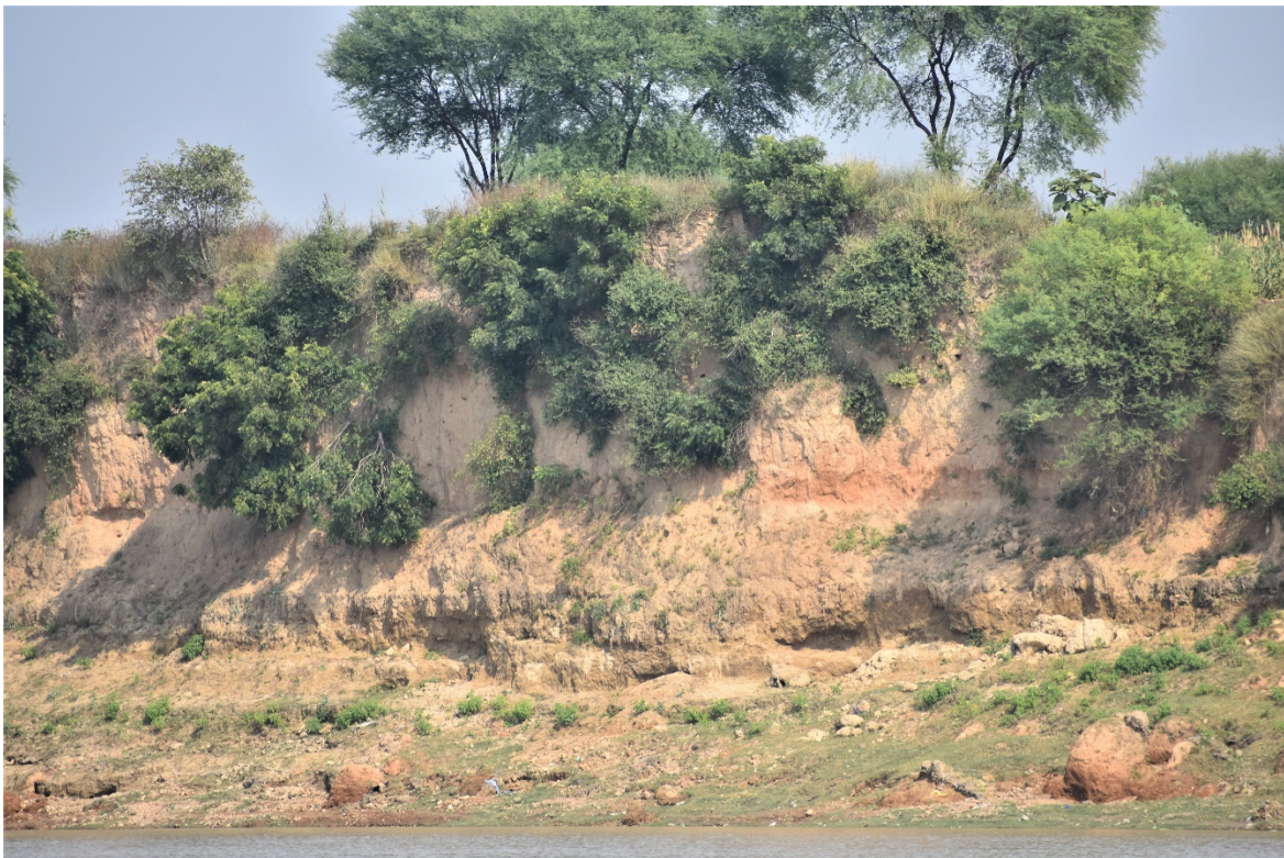
Image 32 : Ganga River Bank Erosion Near Taanda Ghat In Chandauli Distt.
